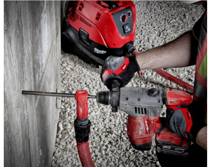
Hollow Vacuum Drill Hole Preparation
